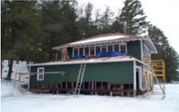
*Gary Kellner repairs rotten roof boards before putting on the new roofing.*
